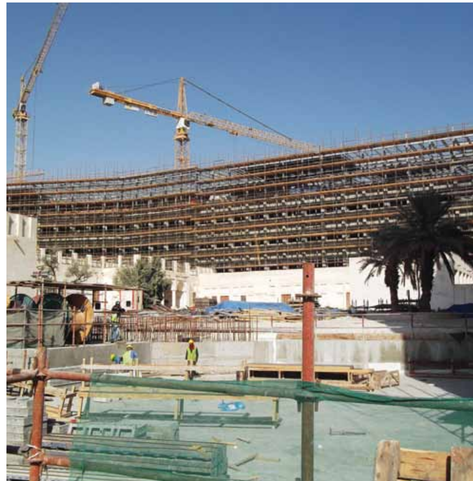
Work being undertaken at the project.
