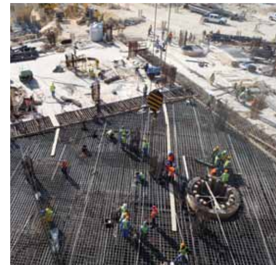
Steel works being installed.
