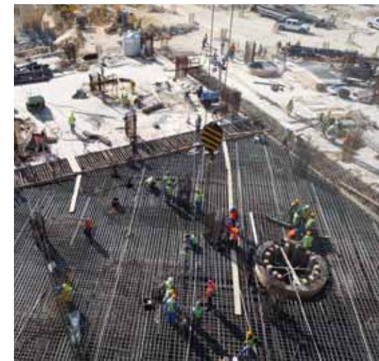
Steel works being installed.
