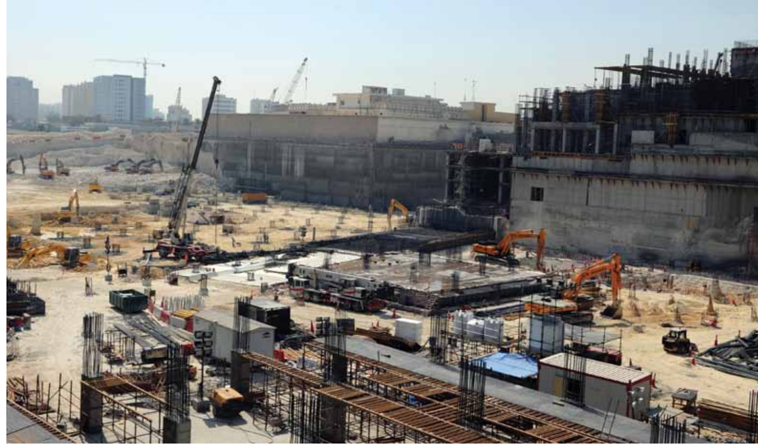
Work on the vast site.
